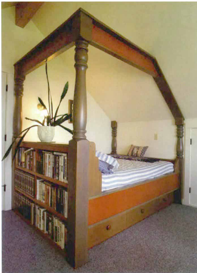
Bookcase as headboard. Vertical-grain Douglas fir, tinted with gray and vermilion, is the predominant material in the captain's bed (above). Cabinets and bookcases flanking the head of the bed in the master suite (facing page) provide storage for bedtime books.
